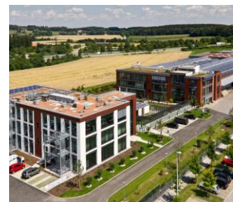
Fig. 1: New company building with 140 kWp (annual) photovoltaic plant
